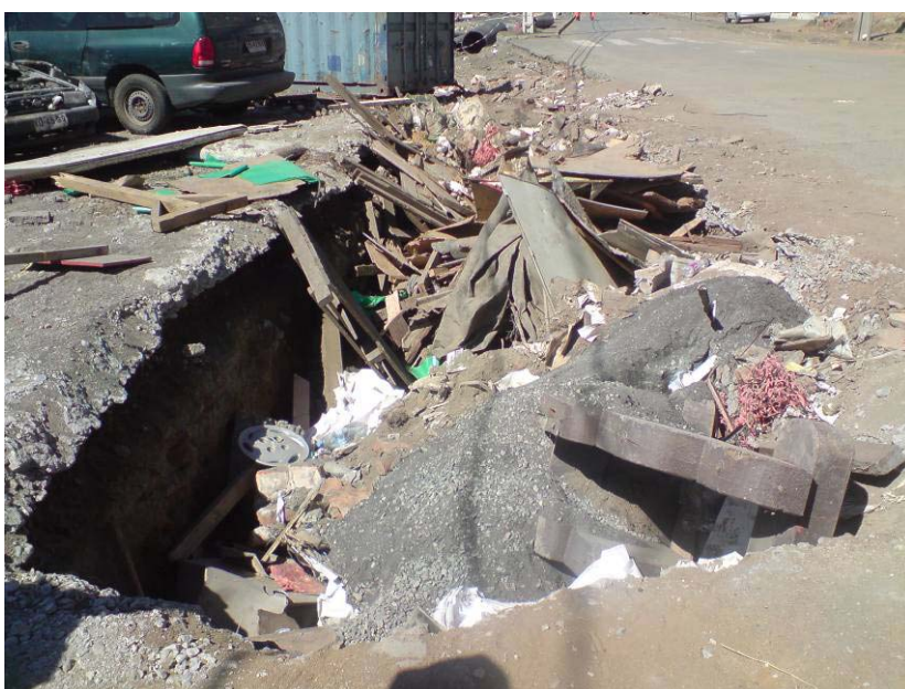
Colector 70, Recolocar tramo de 25ml
